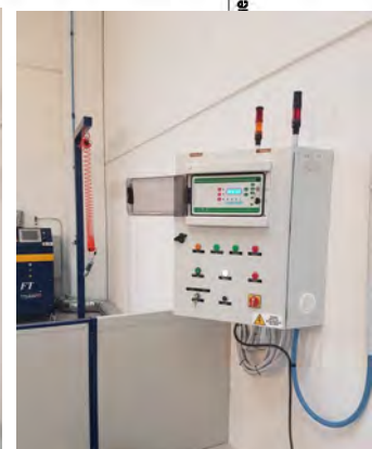
4. Medusa (monitoring and Gas Extraction System)
