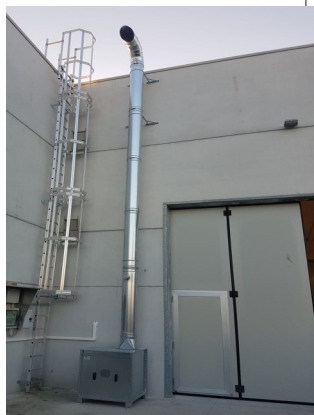
2. Eolo (Fan Unit) Multi Speed ATEX Fan
